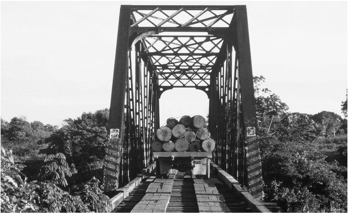
Fig. 6. Another small fraction of the Amazon rain forest on its way to the sawmills of Guajara-Mirim, crossing a tributary of the Madeira on one of the bridges originally built for the railway from Porto Velho and now used for this region's only major road.
